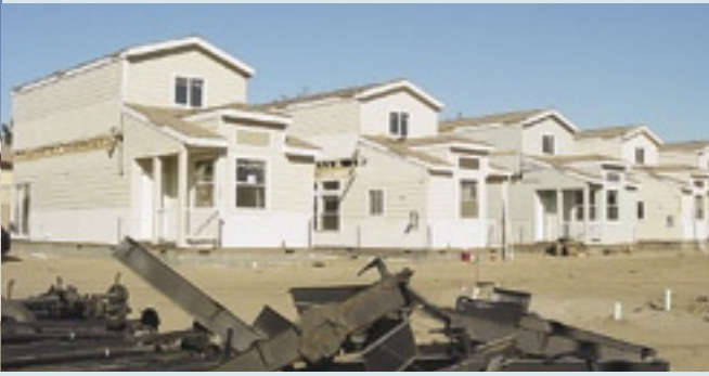
The first five homes were installed with a crane in December 2004. In the foreground are the removed hitches, axles and wheels, some of which will be recycled.
